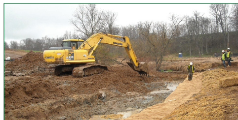
Construction of wetland site
